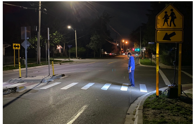
Illuminators on at site #1
