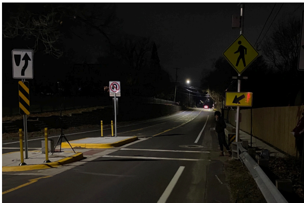
Baseline condition at site #4
