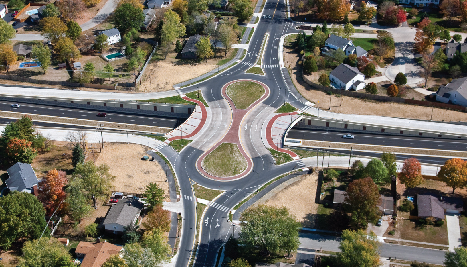
A double-teardrop roundabout on Keystone Parkway in Carmel, Indiana ( American Structurepoint, Inc./Above All Photography )
